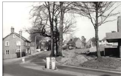
Forest Court under construction, 1962.
